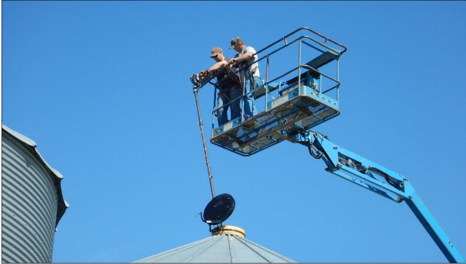
Figure 3. Probe installation process.
