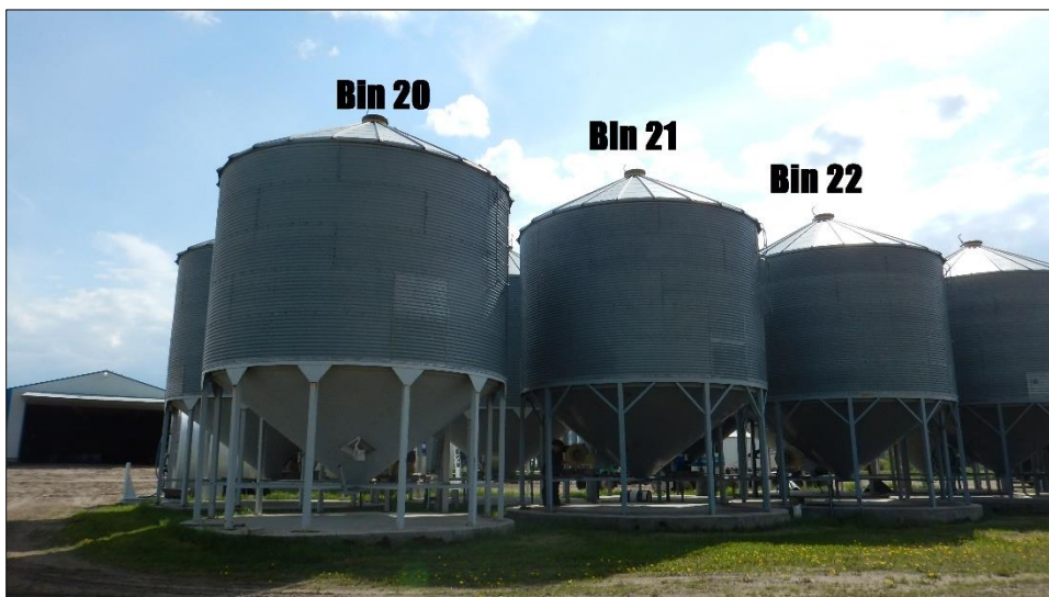
Figure 1. Treatment bin set-up. Bin 20 was the control bin, Bin 21 was aerated in late June, and Bin 22 was partially turned at the beginning of the monitoring period.
