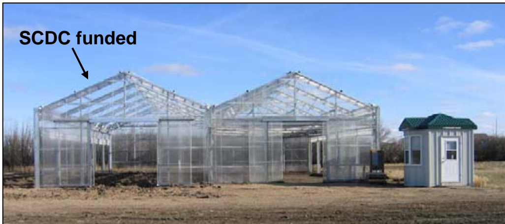
Walls and roof are retractable and plants grow in field soil at ambient temperature and light.
